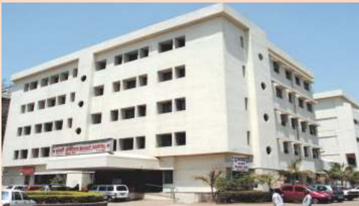
Bharati Hospital, Pune
