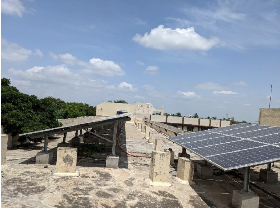
Plate 5: Solar Panel Installation
