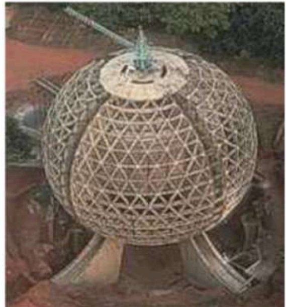
Under construction image of pillars and sphere
