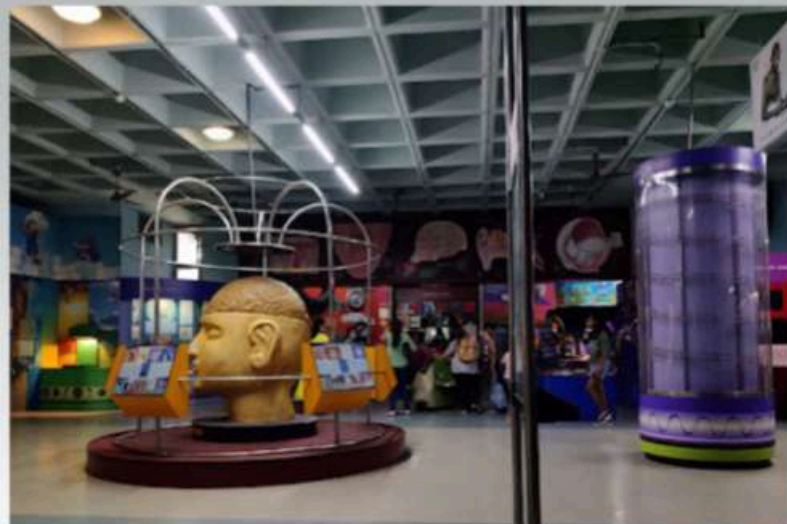
Extensive use of waffle slab to achieve long column free span.
