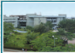
College of Engineering, Pune
