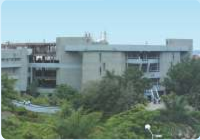
College of Engineering, Pune
